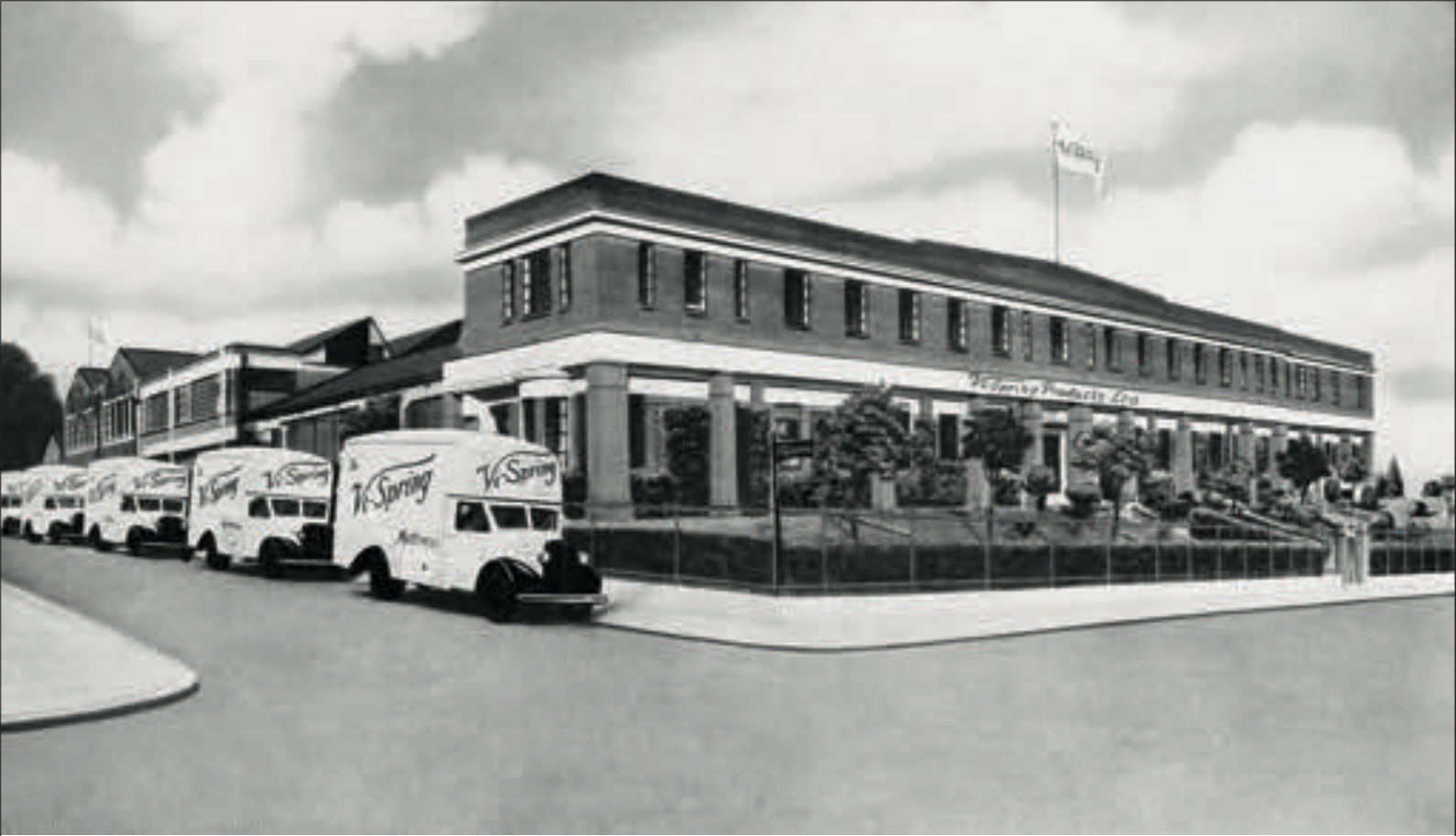
Victoria Road Works, bed production at Willesden Junction, London.
